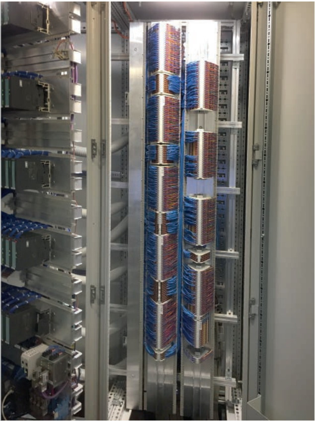
Example of an overhauled control cabinet with the LSC system as a drawer variant with vertical terminals. Practically two wiring levels in one cabinet (Fig.: LÜTZE)
